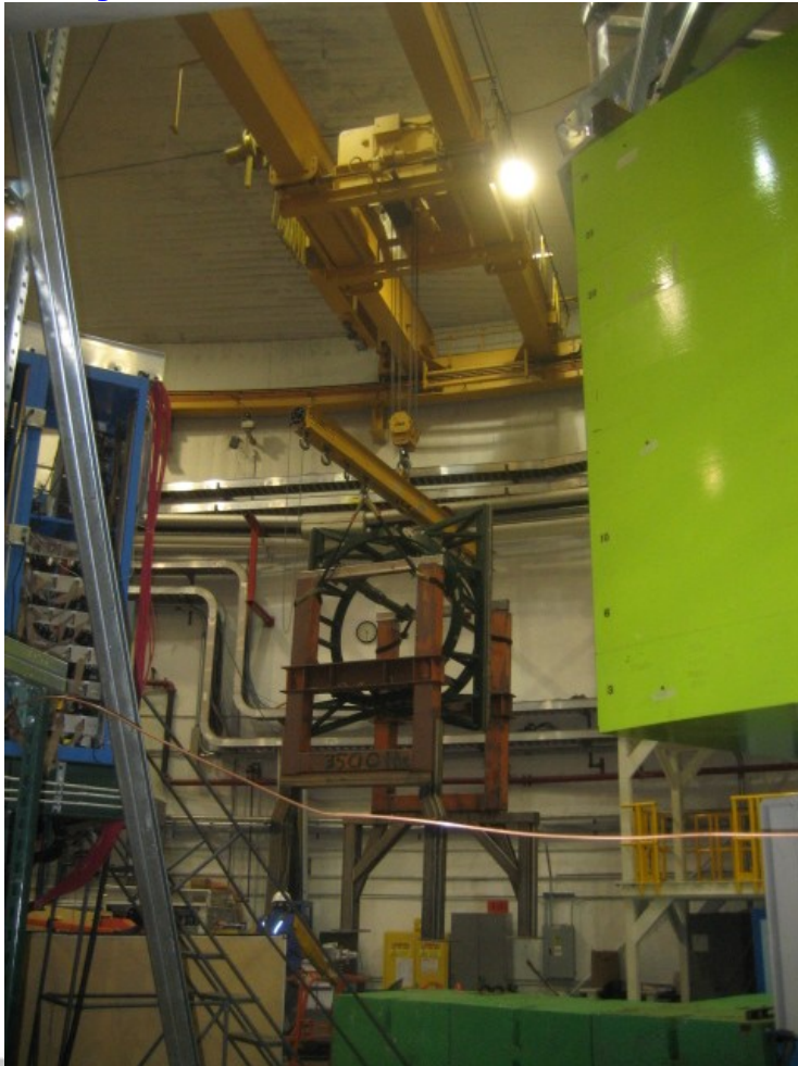
Rotator Superstructure Held by Crane
