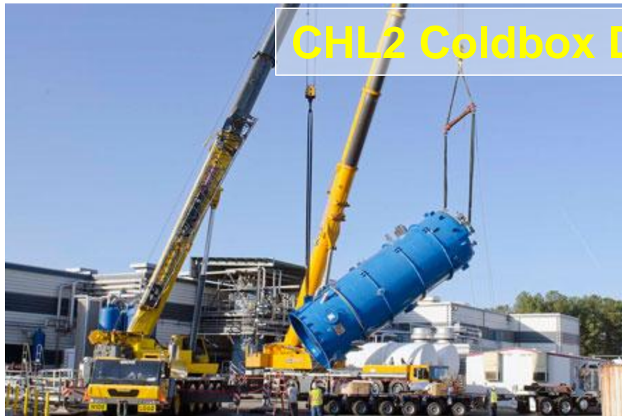
Upper coldbox being erected
