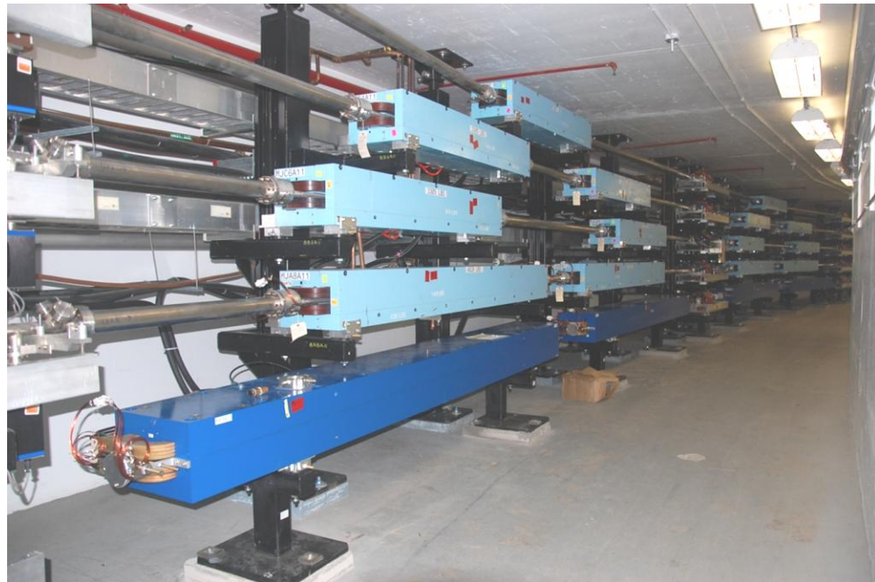
West Arc Refurbished Dipoles & Arc 10 Installation
