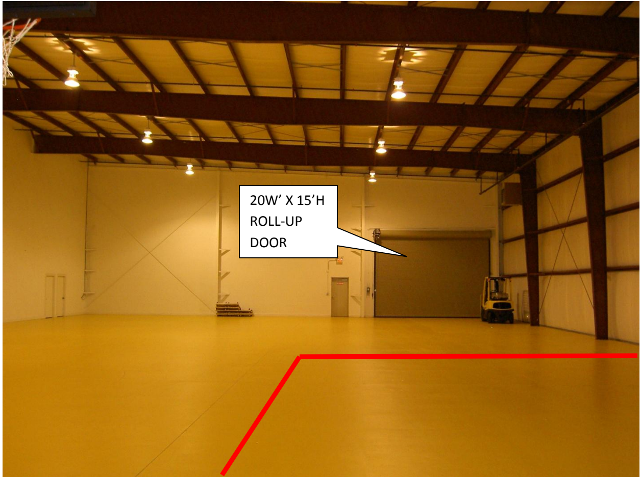
PHOTO TAKEN FROM NORTH WALL LOOKING SOUTH
