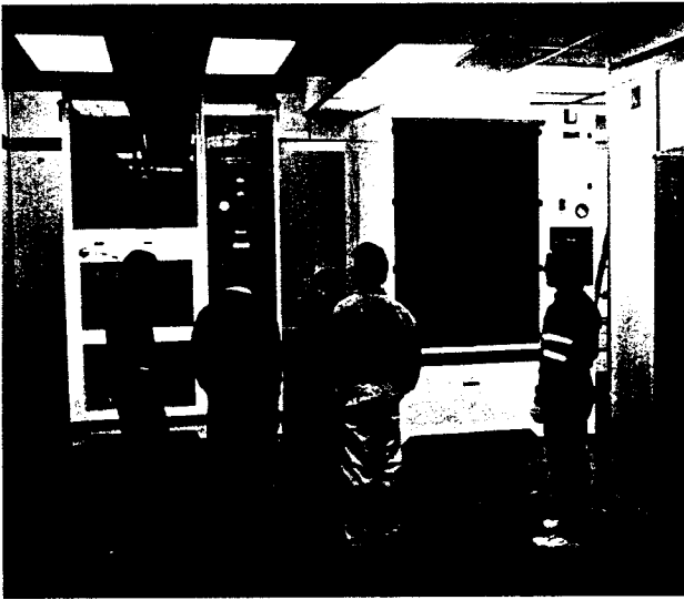
Figure 22: Closed chemistry cabinet (right) and high-pressure rinsing cabinet (left) in the Class 100 production clean room during shutdown for installation.
