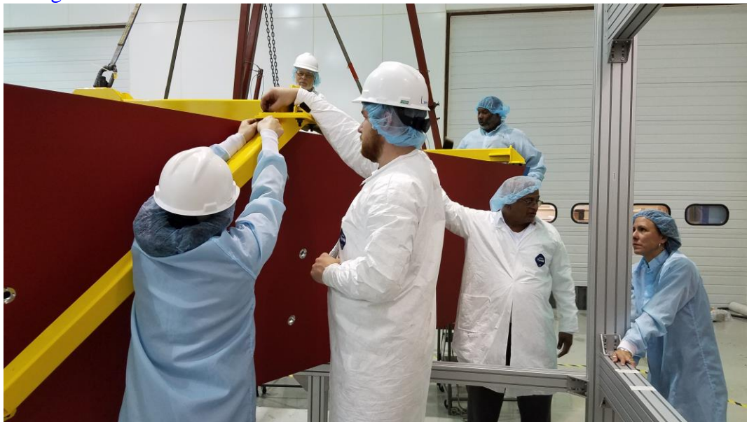
Brian Eng and Tyler Lemon installing lateral arm of stiffening tool
