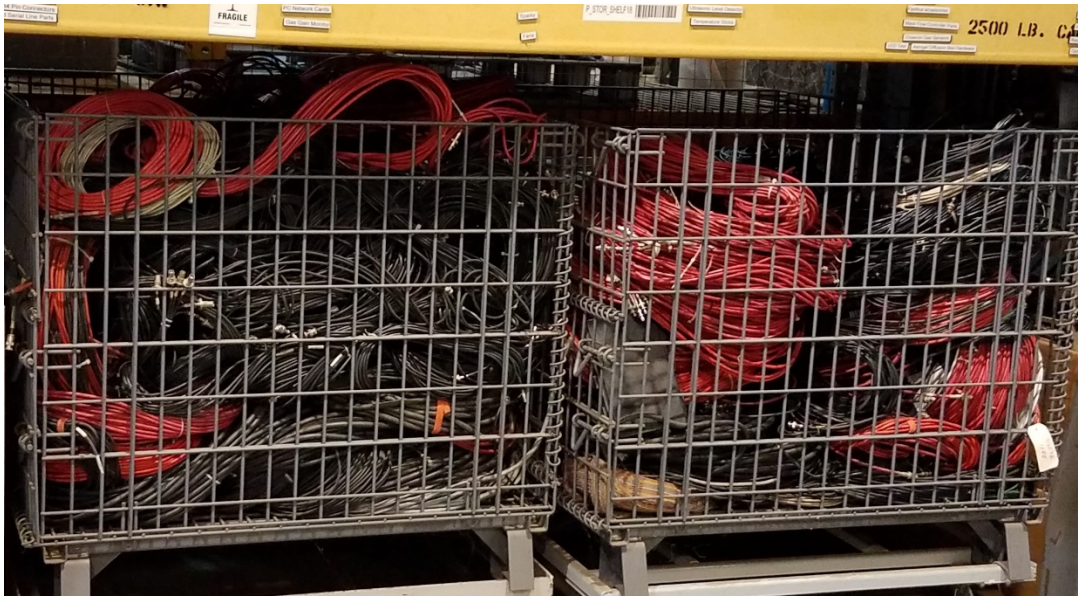
Cables located at Physics storage
