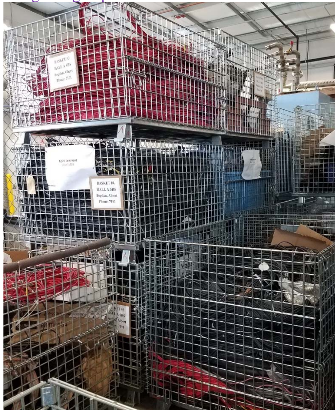
Cables located at ESB building
