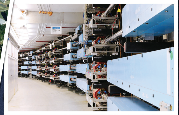
Magnets in a CEBAF beam recirculating arc
