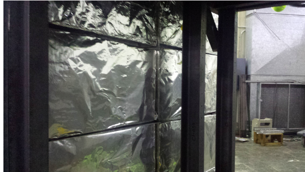
Figure 3: Inside view of C200 mounted insulation panels wrapped in aluminum foil.
