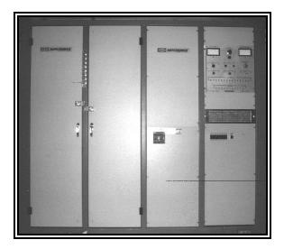
The power supply is housed in a single, welded, steel cabinet approximately 4 bays wide. The dimensions are 72" hi x 48" deep x 90" wide with a weight of around 8,000 pounds. Access to the interior is made via lockable doors and screw-secured panels.
