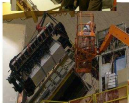
Figure 6: Installation of NaI detector
