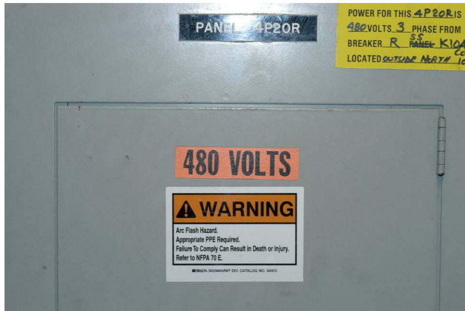
Figure 2-4. Warning label on Panel 4P20R
