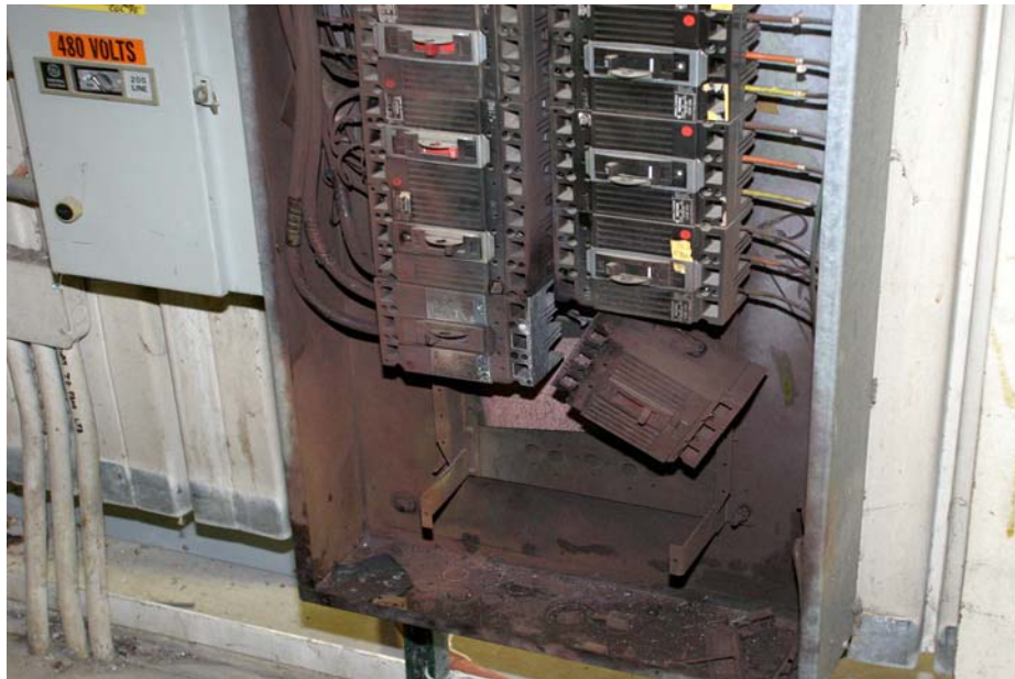
Figures 2-2a and b. Panel 4P20R after the arc flash
