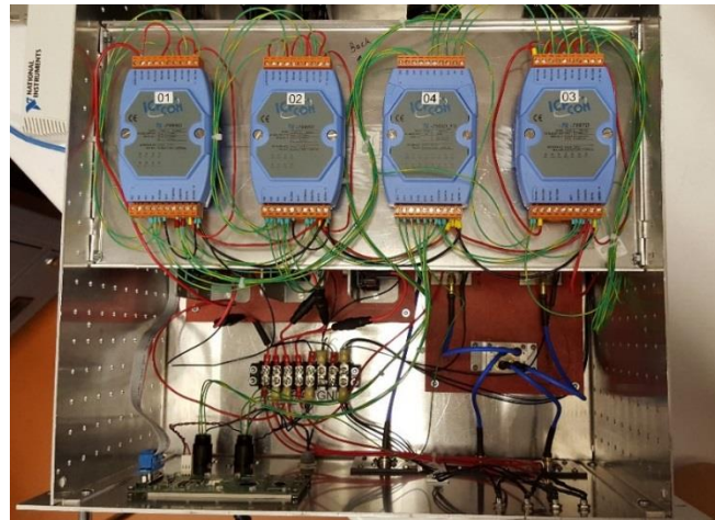
Fabrication 3 rd RF Splitter / Attenuator Box.
