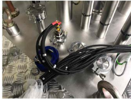
[T sensor check after welding (VBx)]
