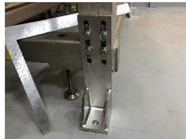
VBx bracket anchoring – initial positioning
