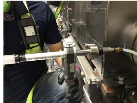
[Extension pipe welding]
