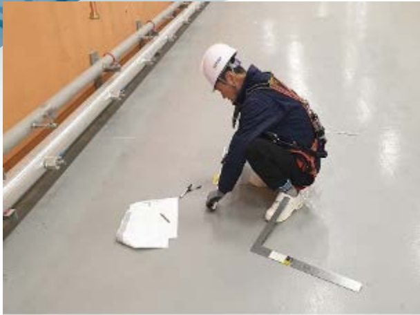
Anchor point marking
