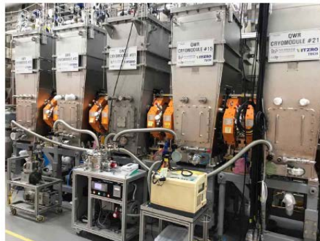
[Evacuation of CM including connection point]
