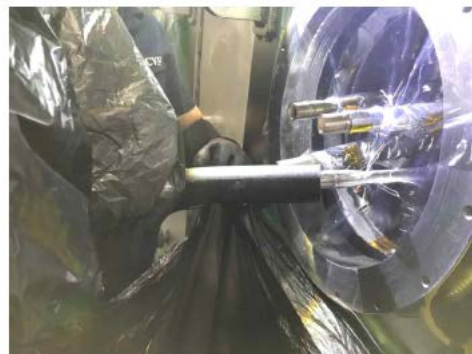
[vacuum cleaning of inner pipe]
