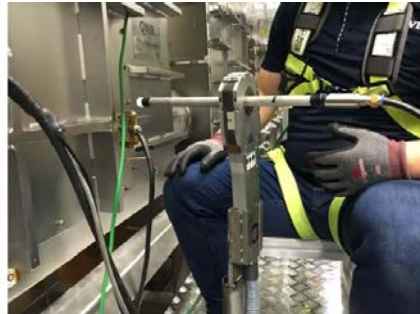
[Welding condition check]
