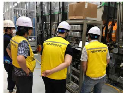
[T sensor signal check before welding]
