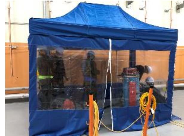
Anchor drilling for Valve Boxes' positioning
