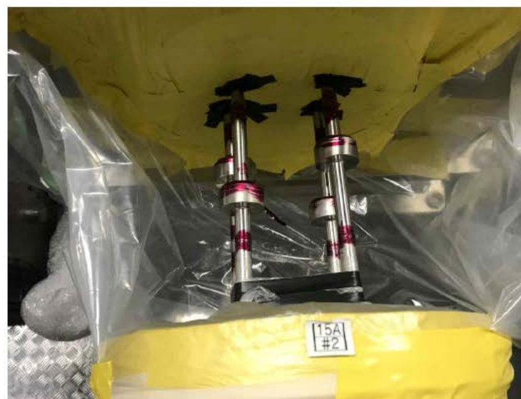
[Application of penetrant ]
