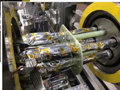
[G-10 Spacer installation]
