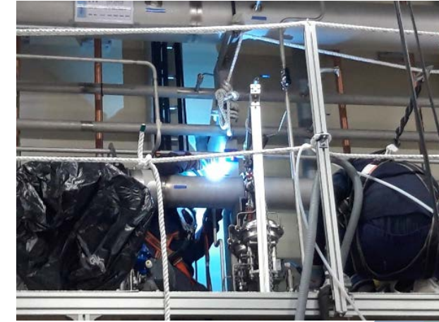
SCL3 warm service line installation
