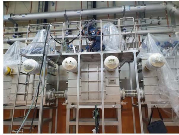
SCL3 warm service line installation
