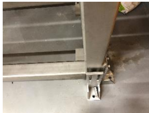
VBx bracket anchoring – initial positioning
