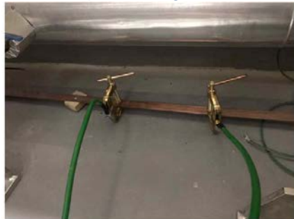
[Ground cable installation on the copper ground]
