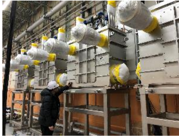
VBx 3 D measurement and alignment
