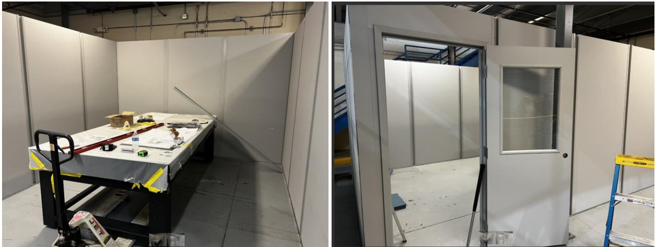
Left: Optical table assembled inside room. Right: Final wall and door of laser-controlled area.
