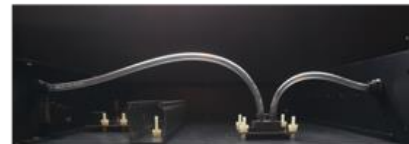
6. Initial gas line installation
