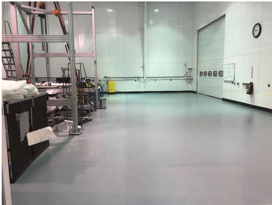
Completed second half of cleanroom floor
